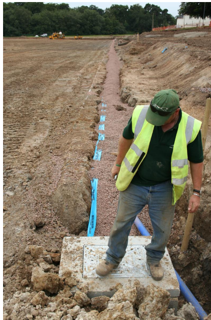
Welshman Steve Evans of White Horse Contractors very much at home while inspecting his 300mm dia cutoff drain.
