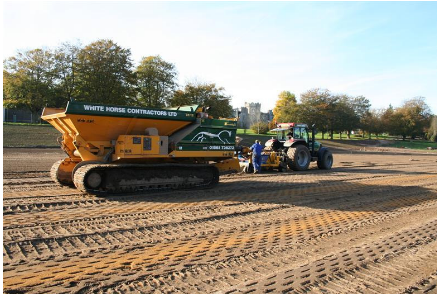
November 2006- Installation of the forced slit drainage system prior to seeding
